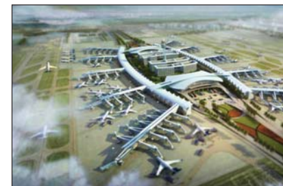
Green Field International Airport
